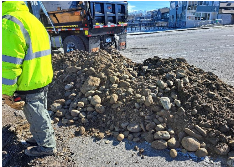
Photo 2: TP-2 excavated material
