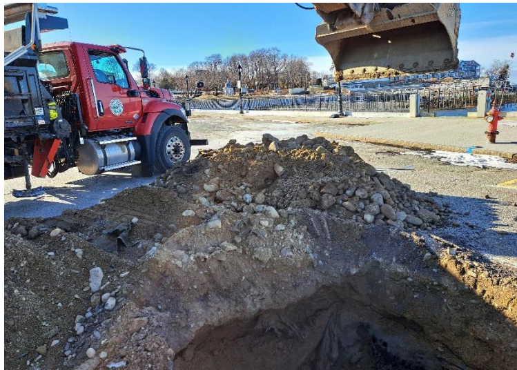
Photo 2: TP-1 excavated material
