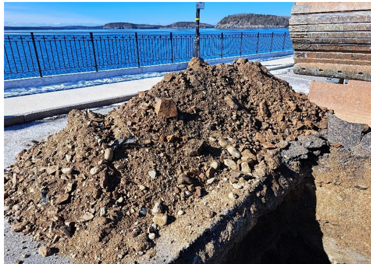
Photo 2: TP-3 excavated material
